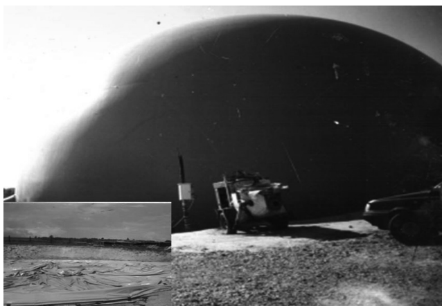
Ill. 5. Air-filled polyvinyl balloon creating the later shape of the burial mound
