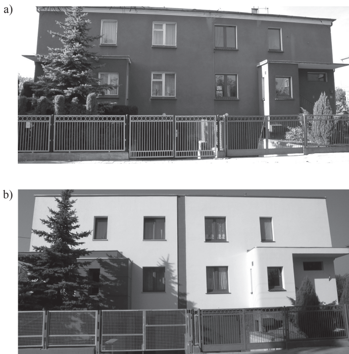
III.8. a) a post-war building before the upgrading, b) the realization of the modernization project; (source: [9])
