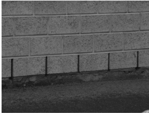
Ill. 9. Plinth of a new building with vent, Martini, Switzerland
