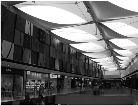
Ill. 5. Shopping Mall Dolce Vita Tejo, designed by Promotorio Architects. Realized and low- E-ETFE-development by Hightex GmbH. Photograph: Hightex GmbH, Bernau
