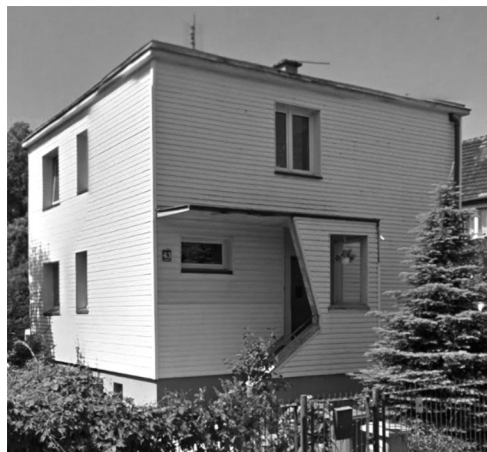
Ill. 4. a) a post-war building covered with siding , b) a post-war house rebuilding by changing a roof shape
