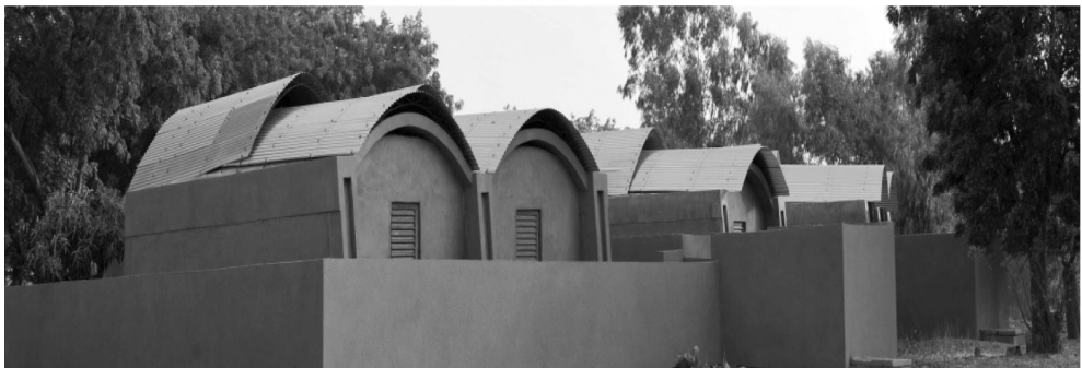
Ill. 13. Teachers housing in Gando, Burkina Faso. Double-layer barrel ventilated roofs (source: [8])
