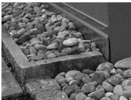
III. 4. Plinth of a new building with the ventilation rim of pebbles, Zurich, Switzerland
