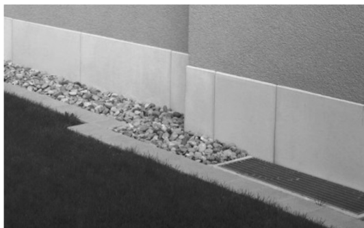
Ill. 2. Sandstone plinth in a new building with a rim of pebbles, Zurich, Switzerland
