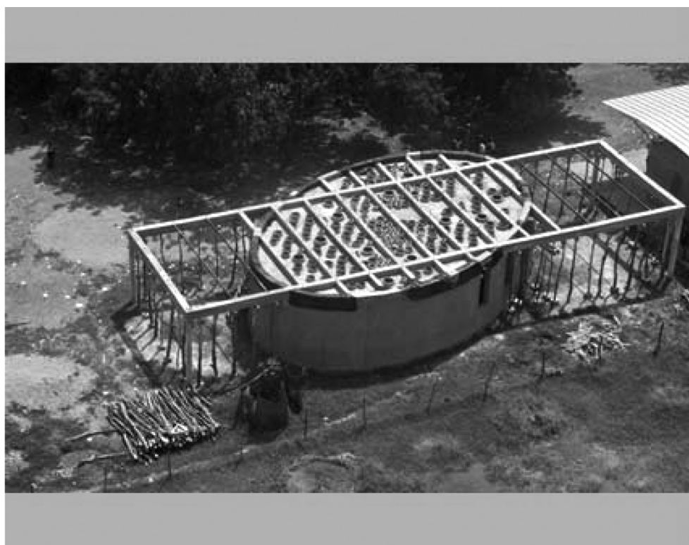
Ill. 14. Library in Gando. Burkina Faso. Top view of a ventilated roof (source: [2])
