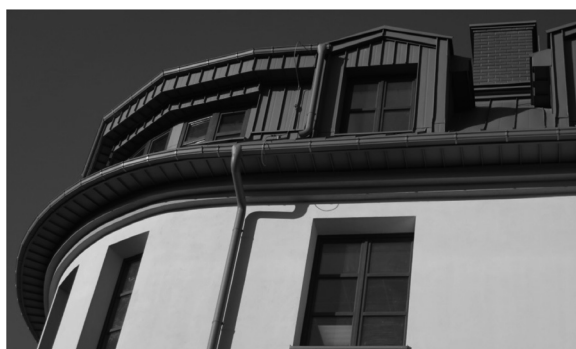
III. 7. Fragment of a part of the roof dormer covered with plate
