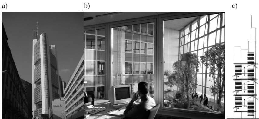
III. 4. Commerzbank Tower exterior facade, interior and ventilation scheme, Frankfurt am Main, Germany, 1997, design: Foster + Partners Ltd Riverside, 22 Hester Road London SW11 4AN (sources: a) author, b, c) [16])
