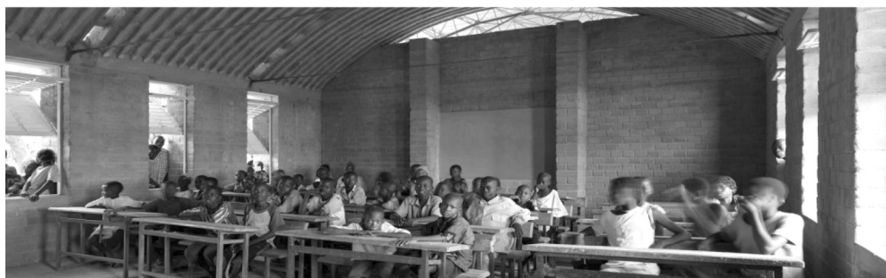
III. 3. School in Gando, Burkina Faso. Classroom with a prominent barrel vault, which contains ventilating holes (source: [1])
