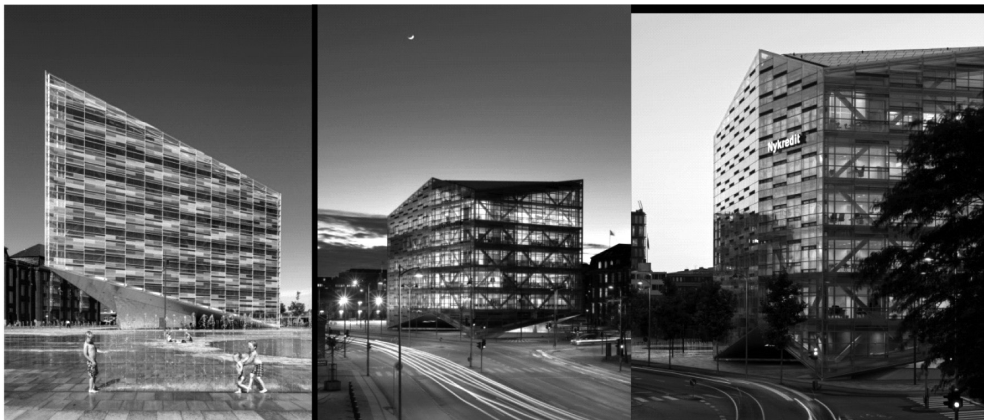
III. 5. External view of the Nykredit bank building facade, which is an integral part of its integrated heating and HVAC system, design: schmidt hammer lassen architects, Aarhus (source: [17])
