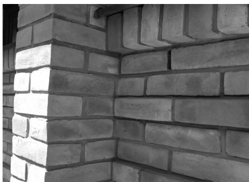
III. 8. New ventilated brick plinth in a monastery, Cracow-Mogila
