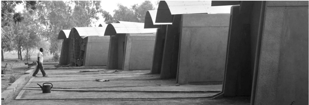
Ill. 12. Teachers housing in Gando Burkina Faso. Visible channels to drain and collect rainwater (source: [8])
