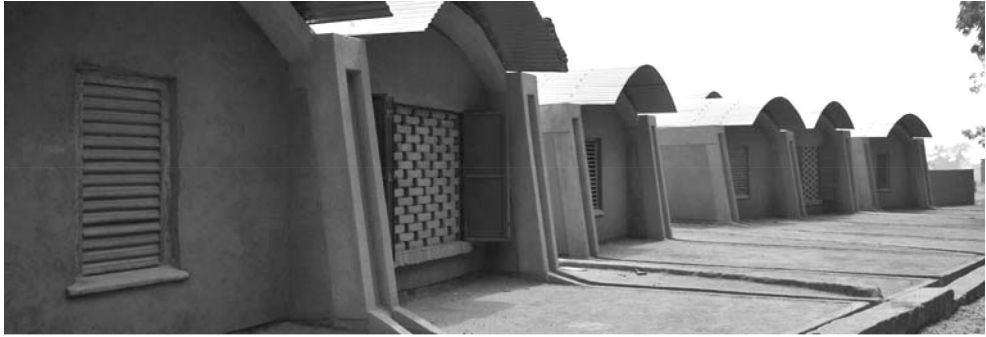
Ill. 11. Teachers housing in Gando, Burkina Faso. Openwork, ventilated front elevation (source: [8])
