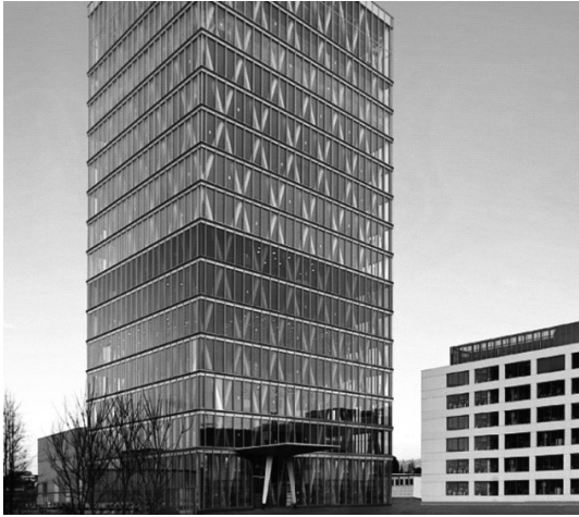
III. 7. Roche Diagnostics AG building in Switzerland, CCF type double-skin facade. Design: Burckhardt + Partner AG, facade design: Josef Gartner and Co, a) facade view (source: [19]), b) horizontal cross-section of the CCF facade: hardened safety glass, laminated (1), aluminum structure (2), facade fastening (3) (source: [18])
