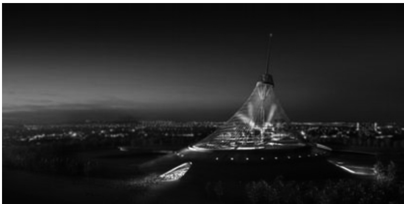
Ill. 4. A general view of the “Khan Shatyr” during the night (source: Conceptual design of Khan Shatyr, Foster and Partners)
