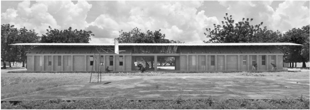
III. 4. School in Gando, Burkina Faso. The facade of the building (source: [1])
