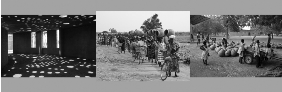
Ill. 15. Library in Gando. Burkina Faso. From left: Main room of the library with a perforated, ventilated roof, rural community carrying clay pots used to build the library (source: [2])
