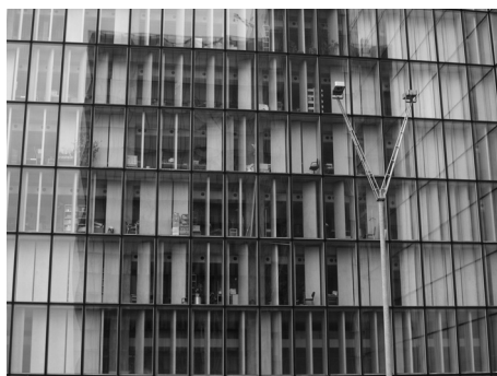
III. 5. The adjustable wooden internal panels (photo by B. Siedlecki)
