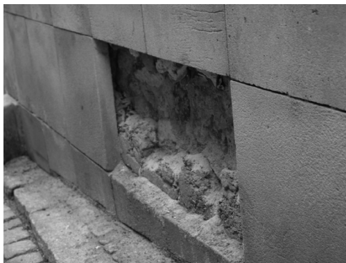
III. 7. Sandstone plinth. Eroded slab due to water vapour condensation, Olomouc, The Czech Republic
