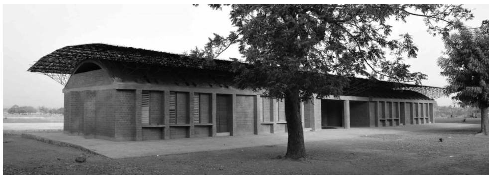
Ill. 7. School in Gando, Burkina Faso. A view of the object (source: [1])
