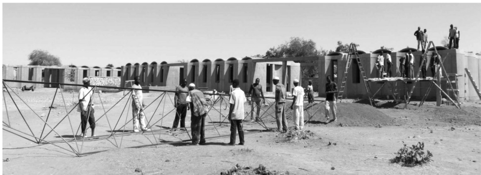
III. 9. Lower secondary school in Gando. Burkina Faso. School building during construction (source: [6])
